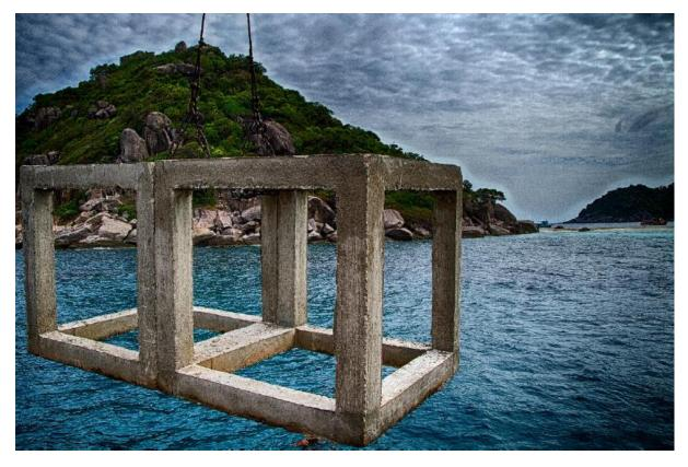
**Figure 1:** One of 140 one tonne concrete cubes deployed in three sites around Koh Tao, Thailand by the Department of Marine and Coastal Resources and the Prince of Songkla University. Photo Andreas Fiskeseth.
