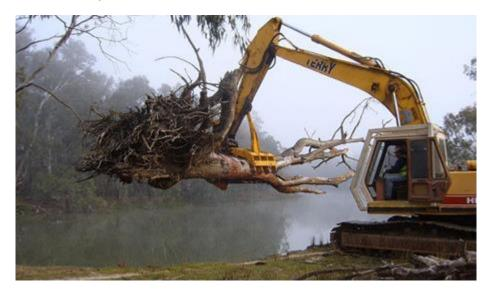
Figure 68: Large snag being installed on the Murray River (Source: Fish Habitat Network).
