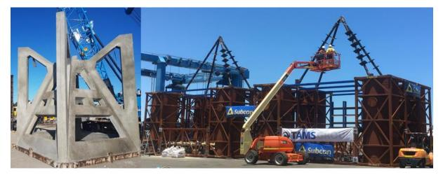
**Figure 19:** Reef Pyramid<sup>TM</sup> (left) and Fish Towers<sup>TM</sup> (right), steel modules constructed and deployed by Subcon (Recfishwest).
