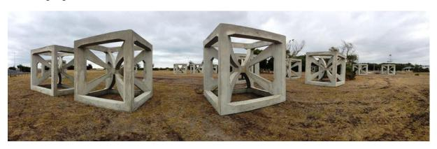
Figure 56: Concrete reef modules awaiting deployment.
