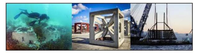
**Figure 55:** Purpose-built artificial reefs, from left to right; Abalone habitat reef, a Fish Box<sup>TM</sup> and the Sydney OAR (http://haejoo.com/).
