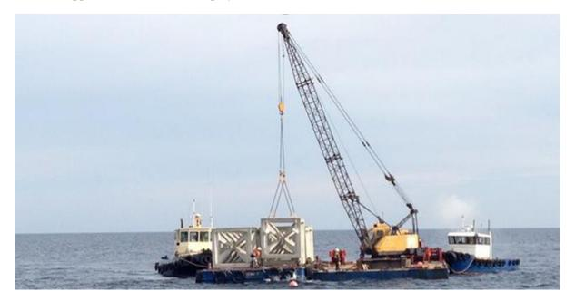
Figure 66: Crane and barge deployment of concrete artificial reef modules in Western Australia.
