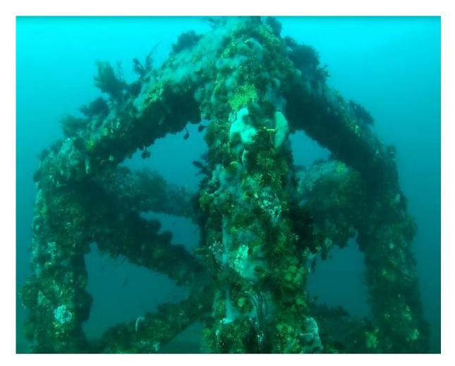
Figure 52: A previously bare surfaced module from the South West Artificial Reef Trial in WA.
