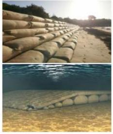
Geotextile bag. Photos from http://www.elcorock.com/ and https://secure.ifai.com/geo/articles/0610\_up1\_reef.html
